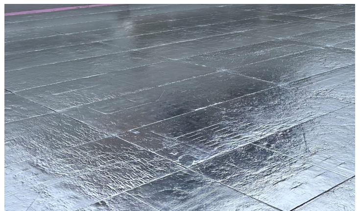
Layer of ADVANC-R ® on a rooftop
